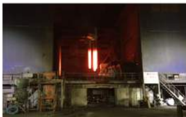
交流电弧炉 Ac Electrical Arc Furnace
